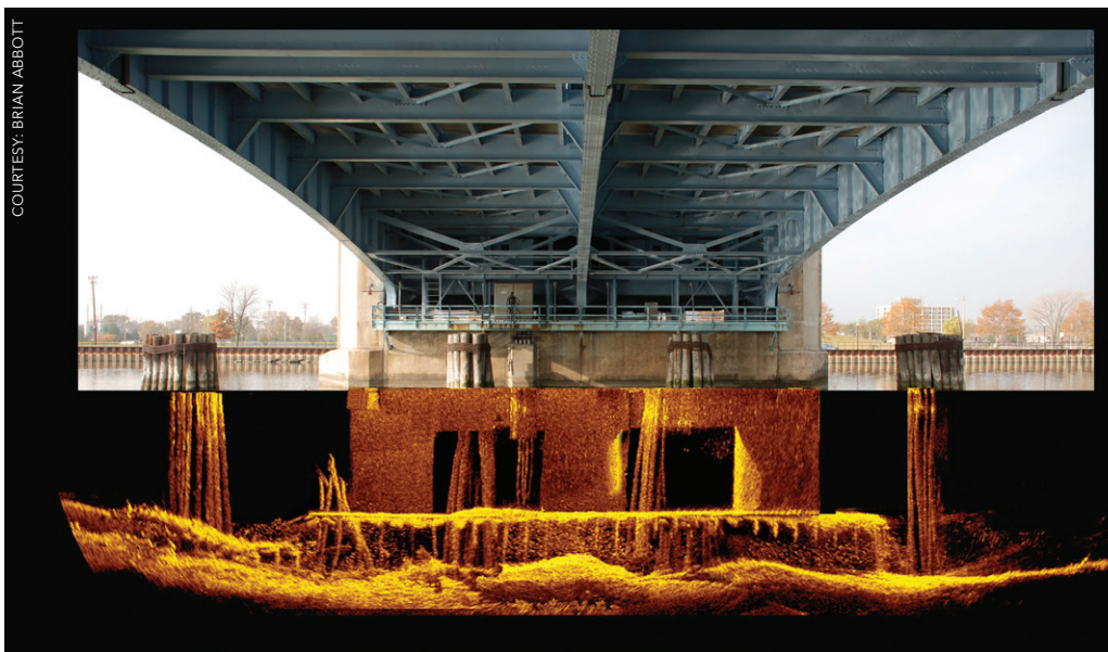
Figure 6. Post-processed sector scan image, showing elevation view of pier.
