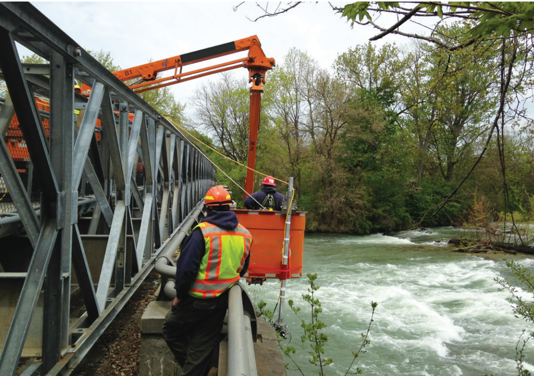
Figure 12. Sonar attached to bucket truck, to evaluate scour during flood conditions.
